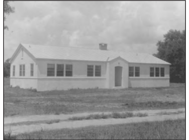
First office building at Ona as seen in 1948, was completed in 1949.
