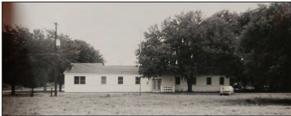
Office building, completed 1969.
