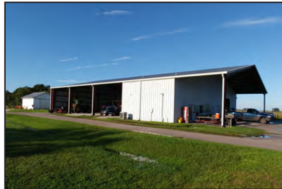
Field Research Facility (shop, equipment barn, farm offices, and breakroom), completed 2008.
