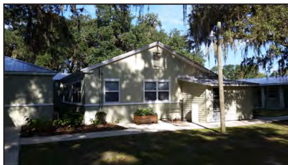
Original office building today.
