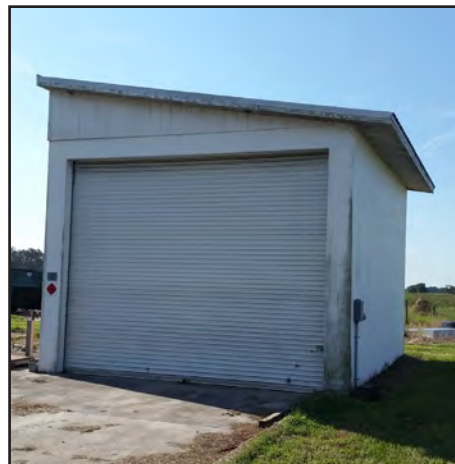
Commodity Feed Building, completed 2009.
