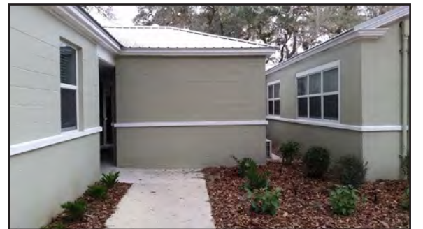
Bathrooms ajoined to the administrative office, completed 2015.
