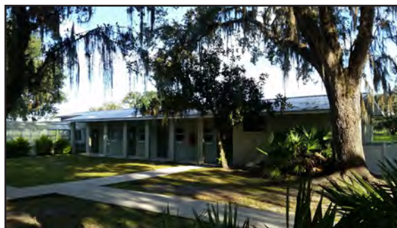
Wildlife and Forage Lab, completed 1964. Soon to be removed for the construction of 2 new labs, offices, and a meeting room.
