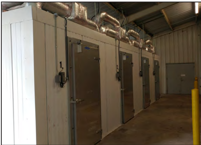
Forage Driers, completed 2016.
