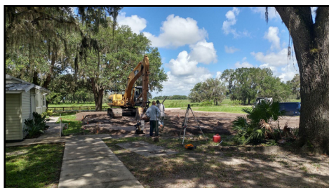
Laying out the foundation.
