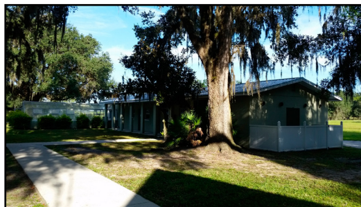
(above) Building before demolition.
