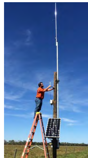
Figure 2: Erecting Tower Gateway and Data-loggers
