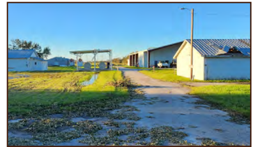
Fuel shed the day after Hurricane Ian, Sept. 30, 2022.
