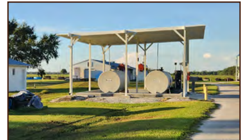
Fuel shed in August 2023.
