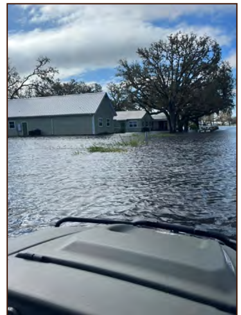
Approaching the Center the day after the storm (9/29). The waters had already receded a foot or more. Photo by Jaime Garzon, one of 3 students onsite for the storm.
